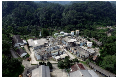
Pongkor Gold Processing Plant
