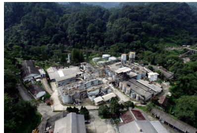
Pongkor Gold Processing Plant
