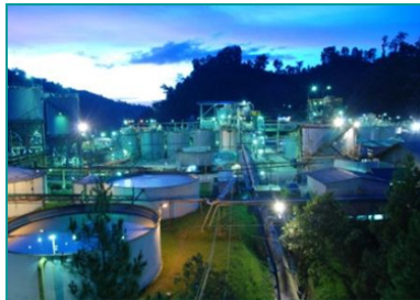
Gold Plant, Pongkor
