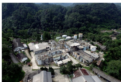
Pongkor Gold Processing Plant
