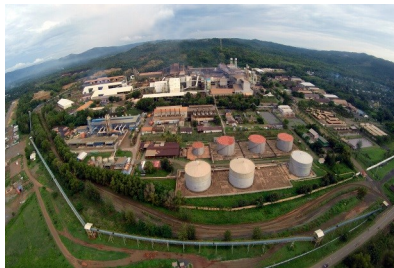
Pomalaa Ferronickel Plant
