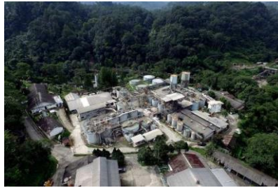
Pongkor Gold Processing Plant
