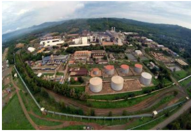
Pomalaa Ferronickel Plant
