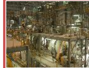
Tayan Chemical Grade Alumina Plant
