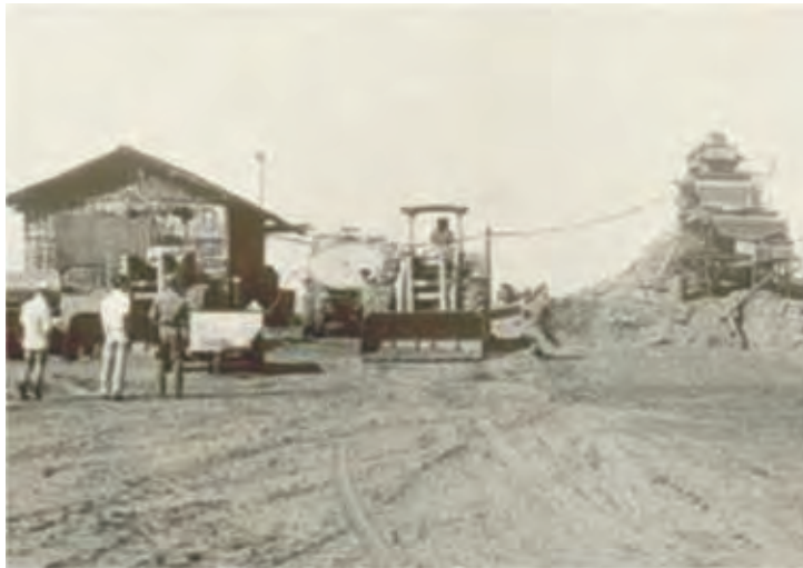
Pay loader prepares to lift the iron sand concentrates.
