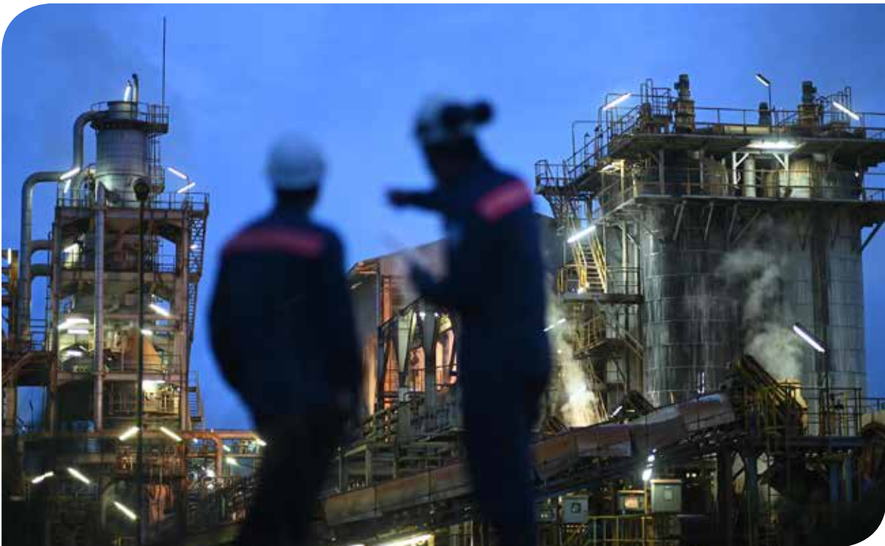
Pabrik chemical grade alumina di Kalimantan Barat. | Chemical Grade Alumina Plant in West Kalimantan.
