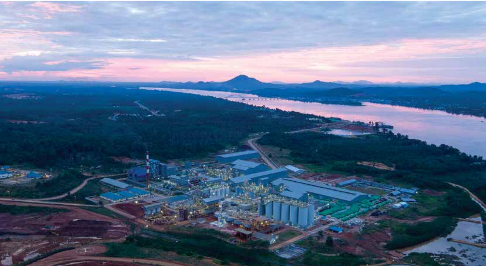
Pabrik Pengolahan Smelter Chemical Grade Alumina di Kabupaten Sanggau, Kalimantan Barat. Chemical Grade Alumina Processing Plant in Sanggau District, West Kalimantan.
