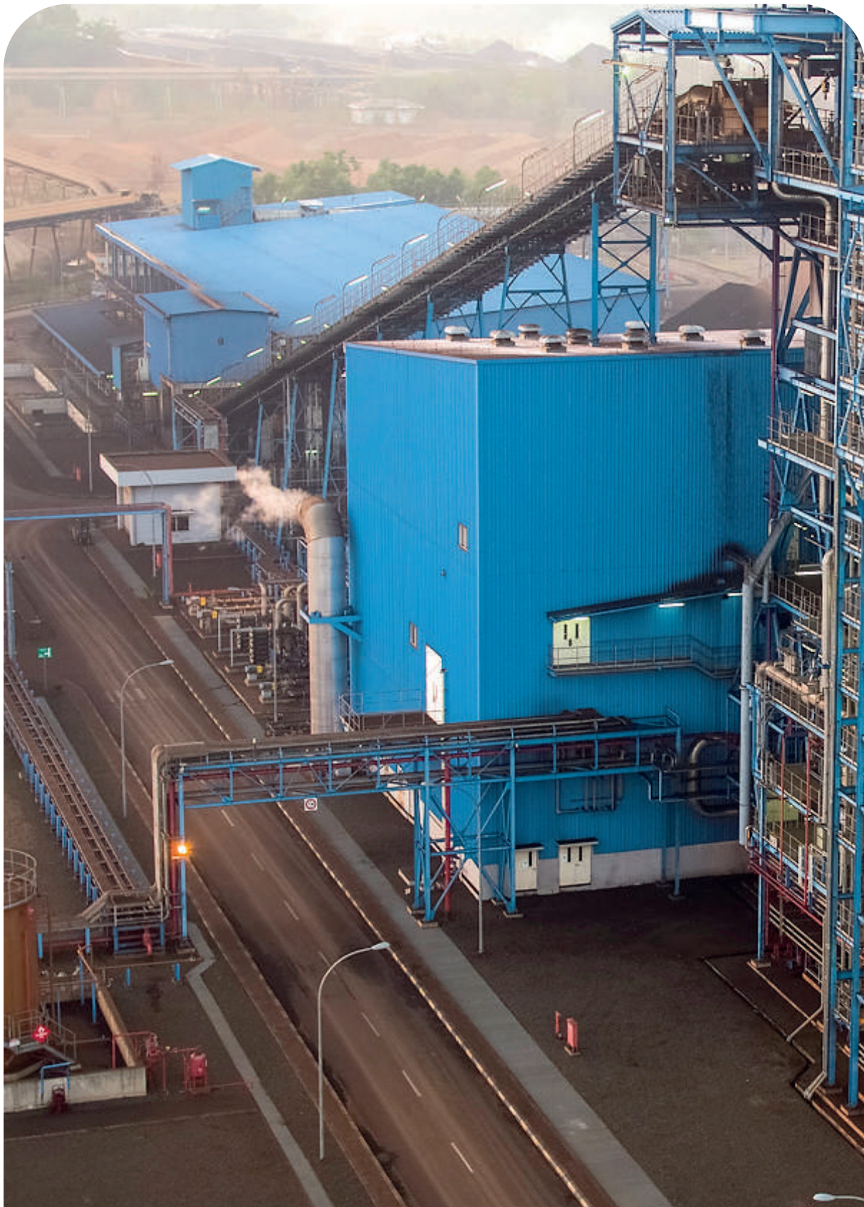
Pembangkit Listrik Tenaga Uap (PLTU) Batu bara UBP Nikel Kolaka, Sulawesi Tenggara Coal-Fired Power Plant at Kolaka Nickel Mining Business Unit, Southeast Sulawesi
