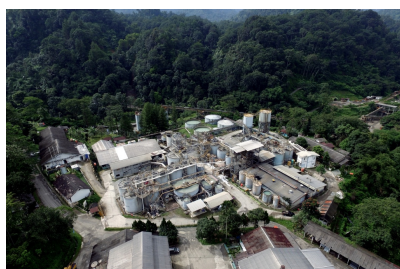
Pongkor Gold Plant
