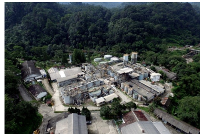
Pongkor Gold Processing Plant
