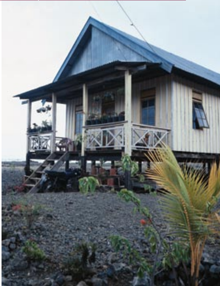
A house near Pomalaa on land reclaimed from the bay using Antam's slag
