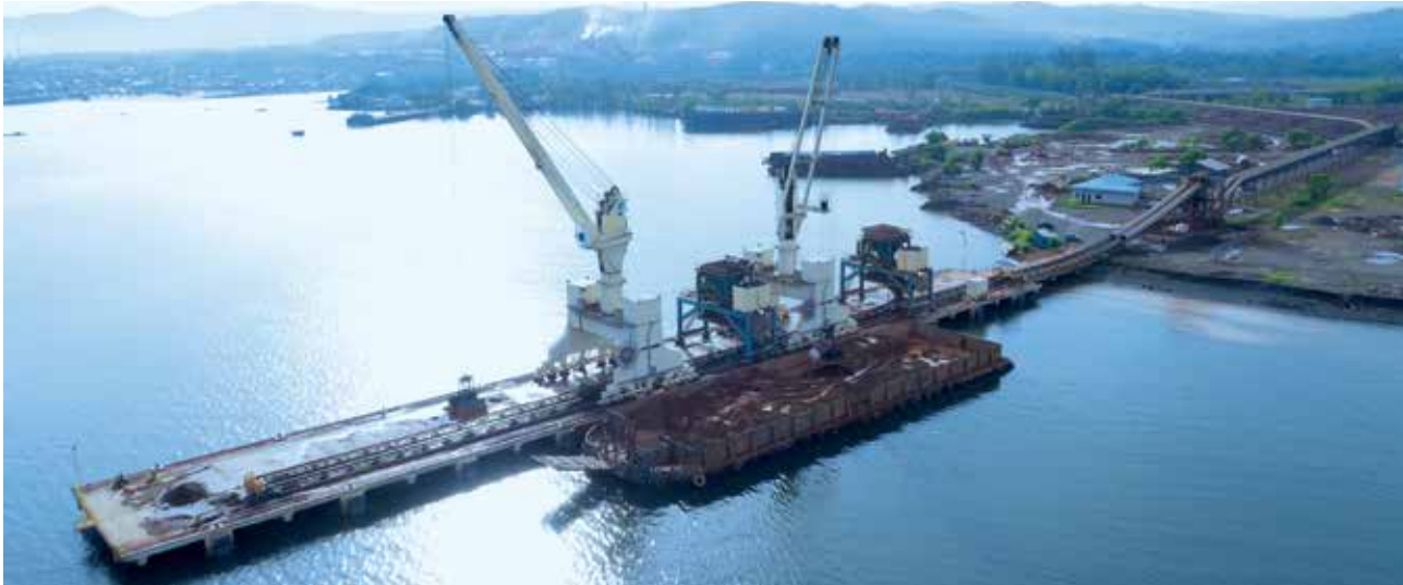
Fasilitas Jetty dan Belt Conveyor ANTAM di Pomalaa ANTAM's Jetty and Belt Conveyor Facility in Pomalaa
