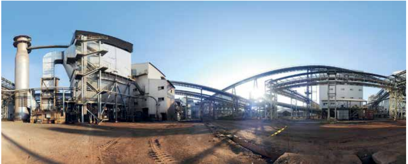
Pabrik Feronikel ANTAM di Pomalaa, Sulawesi Tenggara ANTAM Ferronickel Plant in Pomalaa, Southeast Sulawesi
