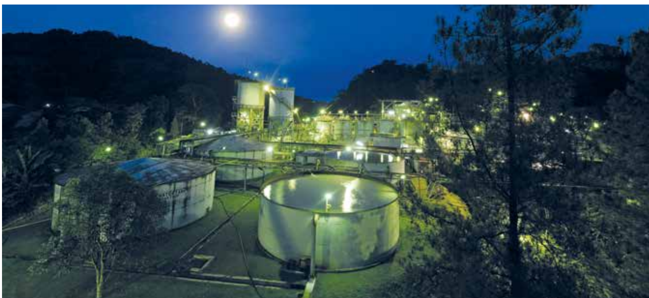
Pabrik Pengolahan Emas di Pongkor Pongkor Gold Processing Plant
