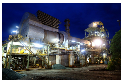
Pomalaa Ferronickel Plant
