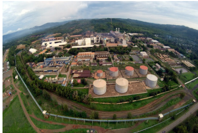
Pomalaa Ferronickel Plant
