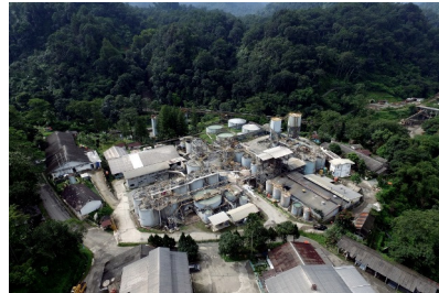
Pongkor Gold Processing Plant
