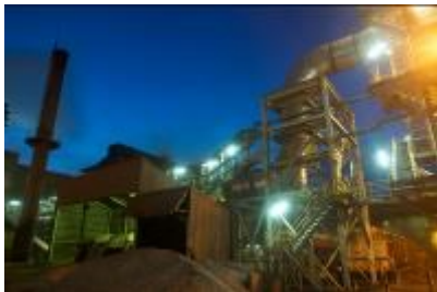
Pomalaa Ferronickel Plant
