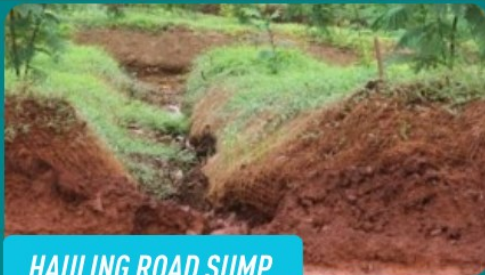
HAULING ROAD SUMP
